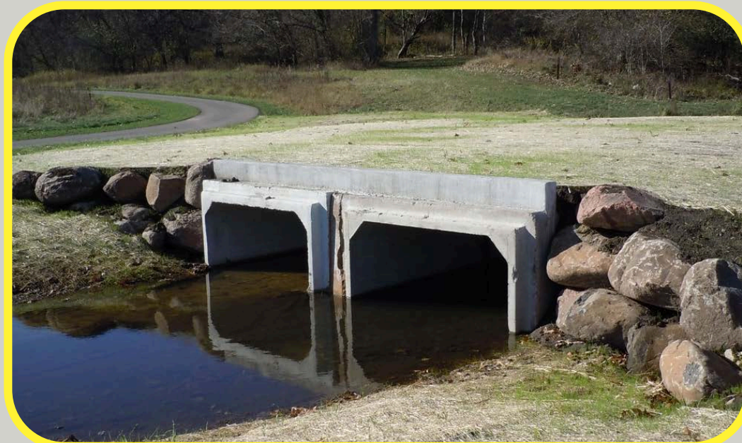
3a -Culverts at sanitary access path crossing - allows consistent and safer vector access
